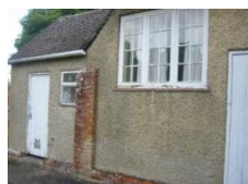
New doors and new lower windows
