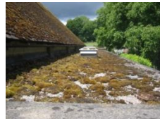
Flat roof repairs and new insulation
