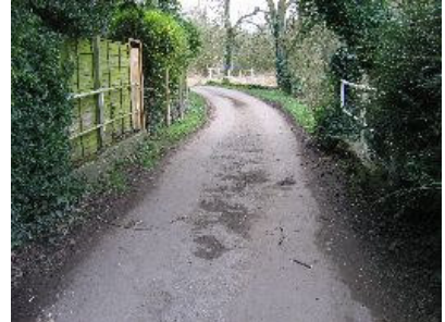
Photos of existing bridge
